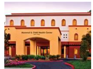
SAN YSIDRO HEALTH CENTER
