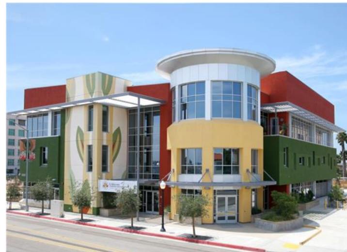
LEED Certified Gold Health Center, opened 2010
