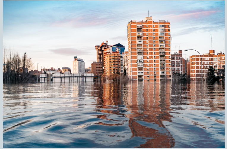
Flooding of public housing units, Photo courtesy JJFarquitectos.
